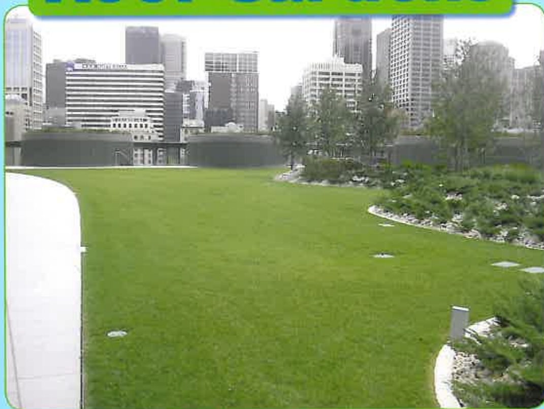
Fantastic visual effect from Hydrocell RG 30 used as the base and Hydrocell lightweight soil as overlay for the garden at Freshwater Place in Melbourne.
