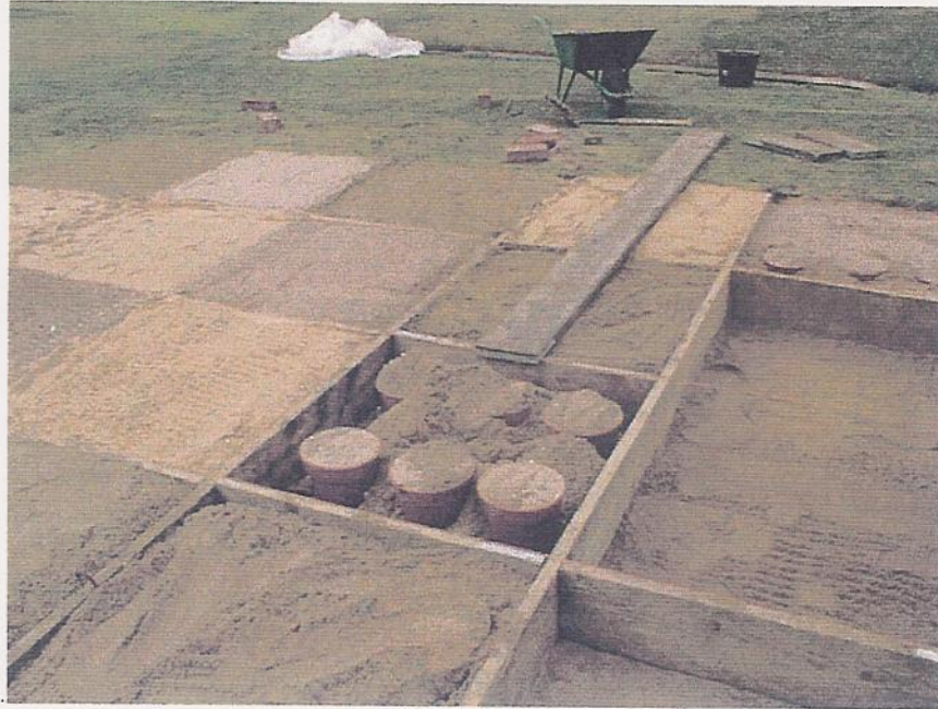
PLATE 1 Installation of the lysimeter pots during the trial construction
